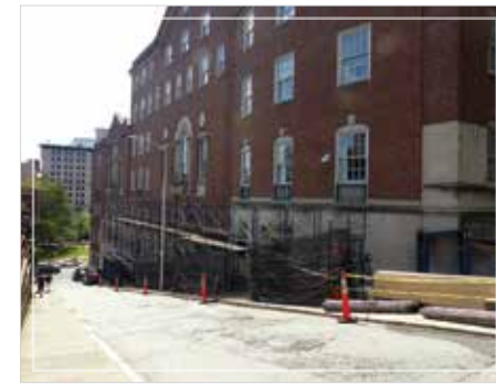
Repairs to the façade at the Licht Judicial Complex.
